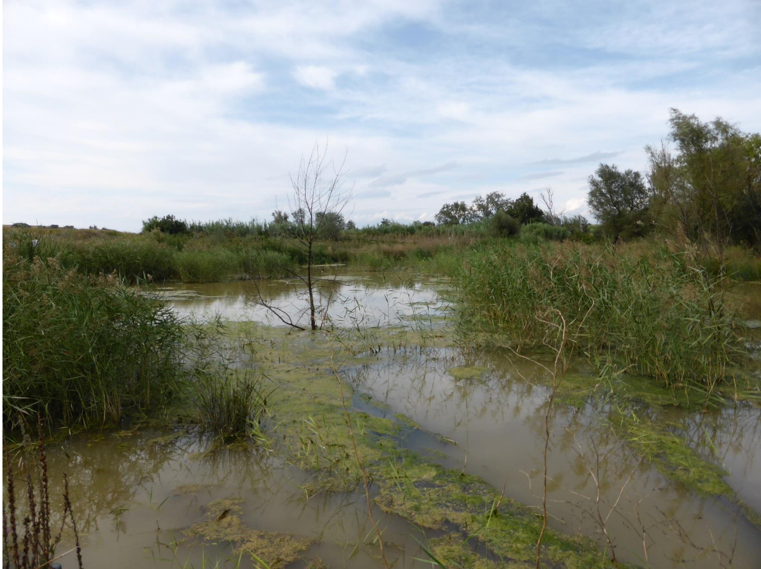
Constructed wetland for treatment of agricultural drainage near Padova, Italy.
